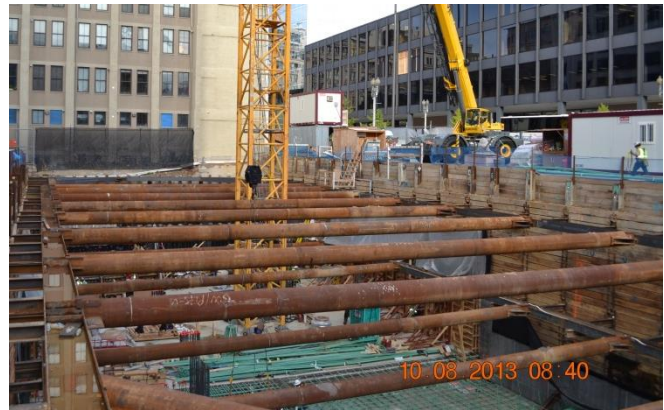
Figure 1. Installation of Mat Slab
